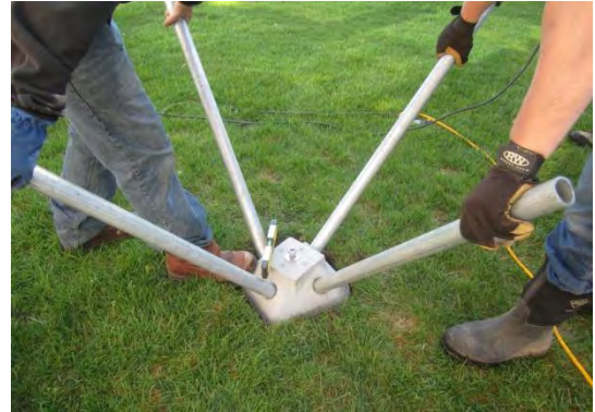
Figure 6. Setting Pins and Leveling Concrete Head
