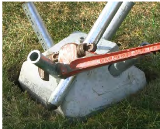
Figure 8. Jacking Method for Pin Removal
