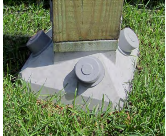
Figure 9. Completed Installation with Pin Caps
