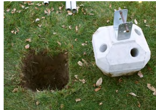
Figure 5. Tapered Hole for Concrete Head
