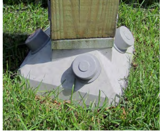
Figure 9. Completed Installation with Pin Caps
