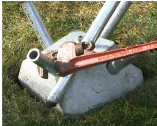
Figure 8. Jacking Method for Pin Removal
